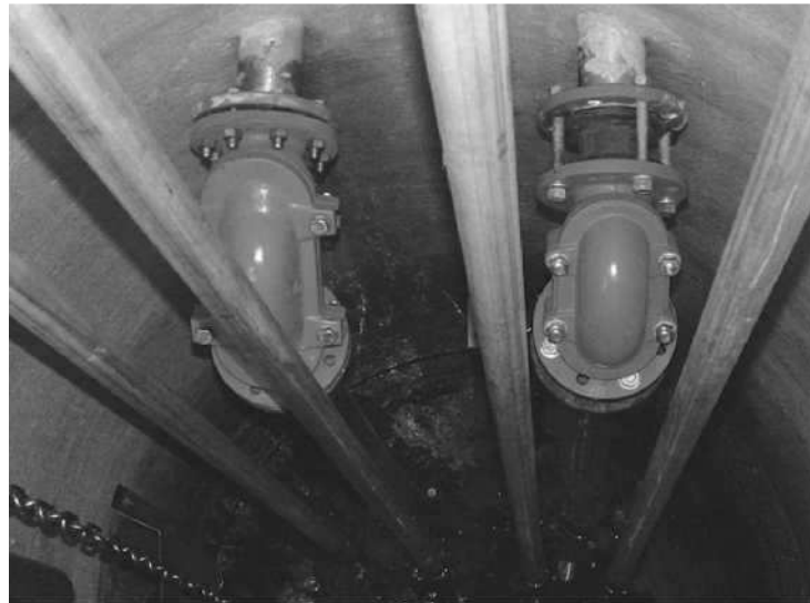
Pic. 1. SZUSTER system valves: on the left – a valve with a long cover (previous construction model); on the right – new valve in a short cover.
